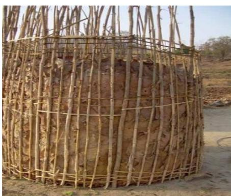
**Fig 4: Structure of Beris using Bamboo**
