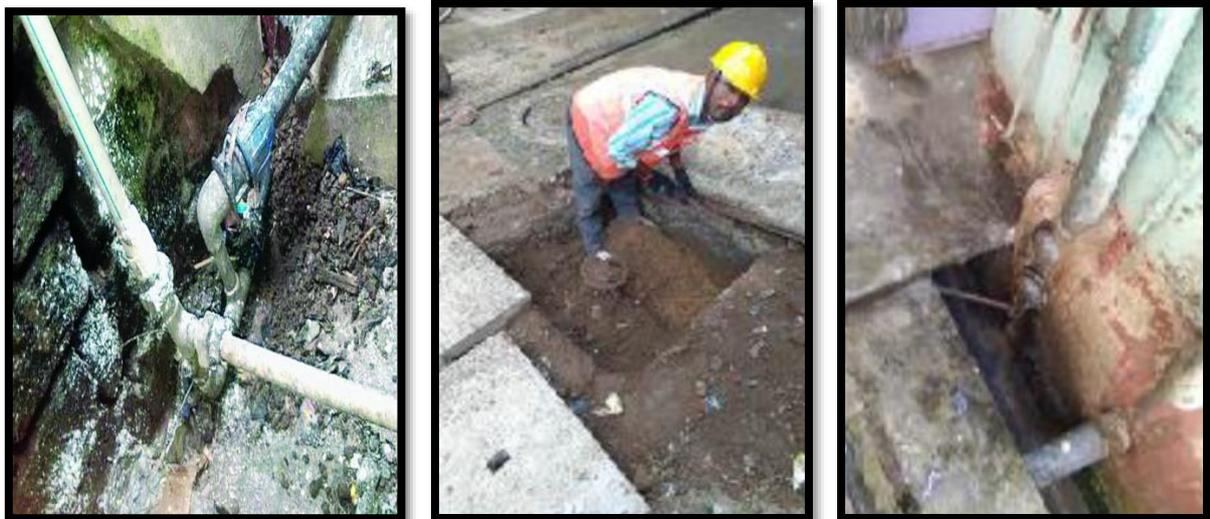
**Fig: 8 Water pipelines leakage and connection stealing (Quarterly newsletter from NCDC)**
